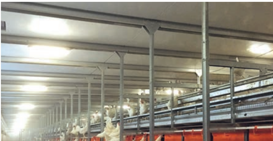
The smooth, white surface of the plastic boards allows the fresh air to flow crosswise through the barn without obstructions and also increases brightness in the lower level
